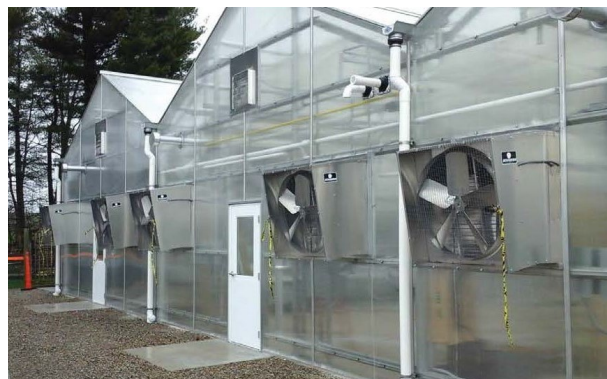
Photo of ATI Greenhouse Replacement: The new 5,447-SF collage level educational greenhouse range at ATI, comprised of three 1,440-SF compartments, replaces 2,343-SF of poly-tube greenhouse space. Each of the 60'x24' compartments, with a BL1-P Bio-Safety level, addresses either Propagation, Production or Management disciplines.
